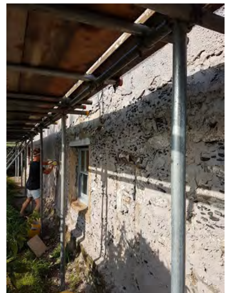
Chris, showing work in progress, pointing the walls with lime © Sue Bletcher
