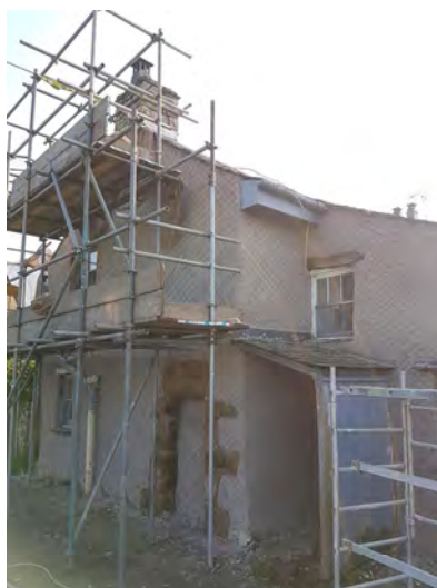
Chris, showing work in progress, pointing the walls with lime © Sue Bletcher
