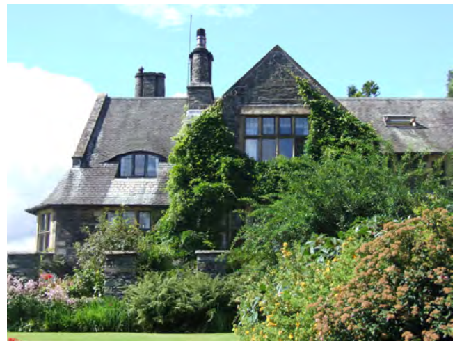
Cragwood rooflines © Mike Turner
