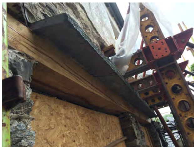
New timber in place © Sue Bletcher
