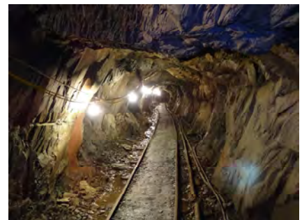
The entrance tunnel
